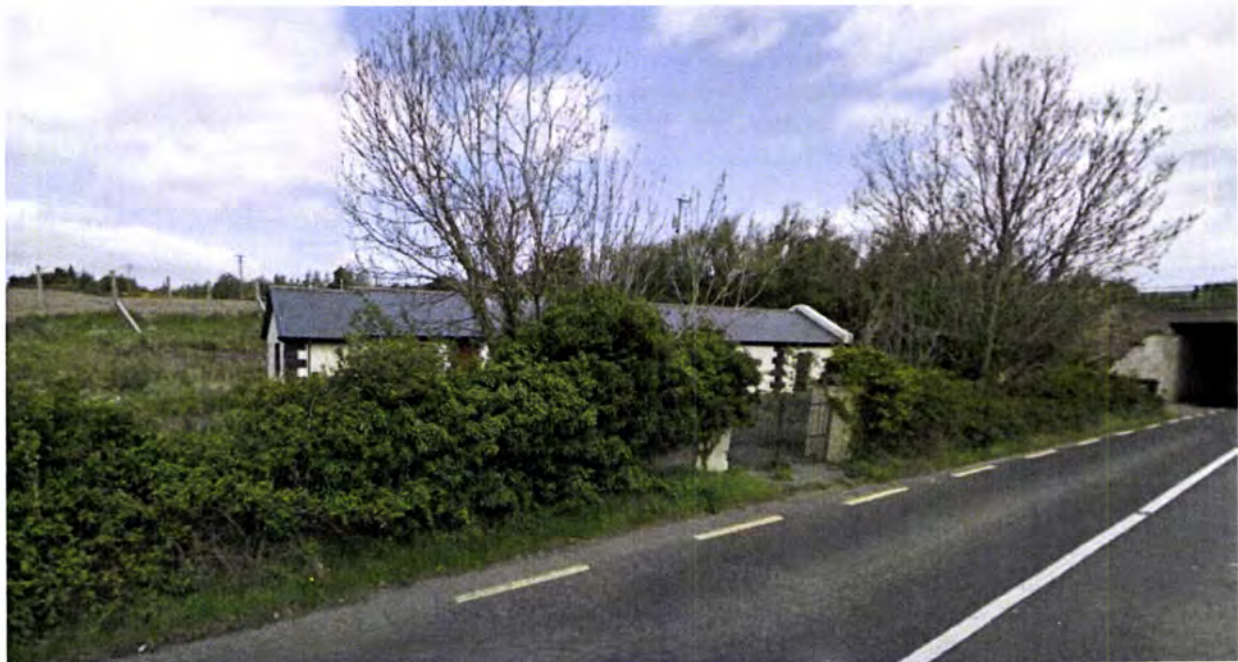
Photograph 1: The land has accommodated a building for circa two hundred years, with this structure having formerly been used as a house with an attached forge.
